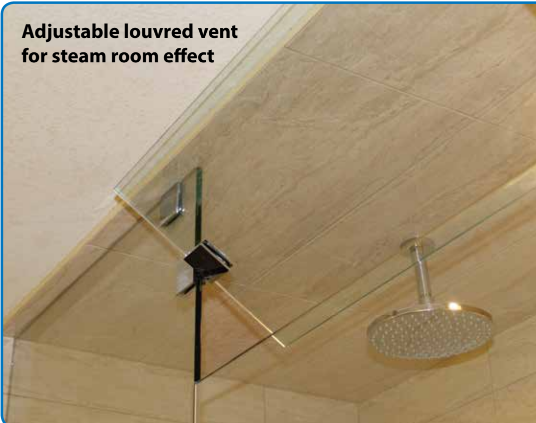
Shower with frameless glass, overhead rain-head, and sliding bar for shower-head height adjustment
